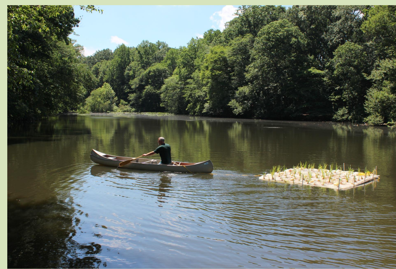
Towing artificial floating wetland to anchoring location.
