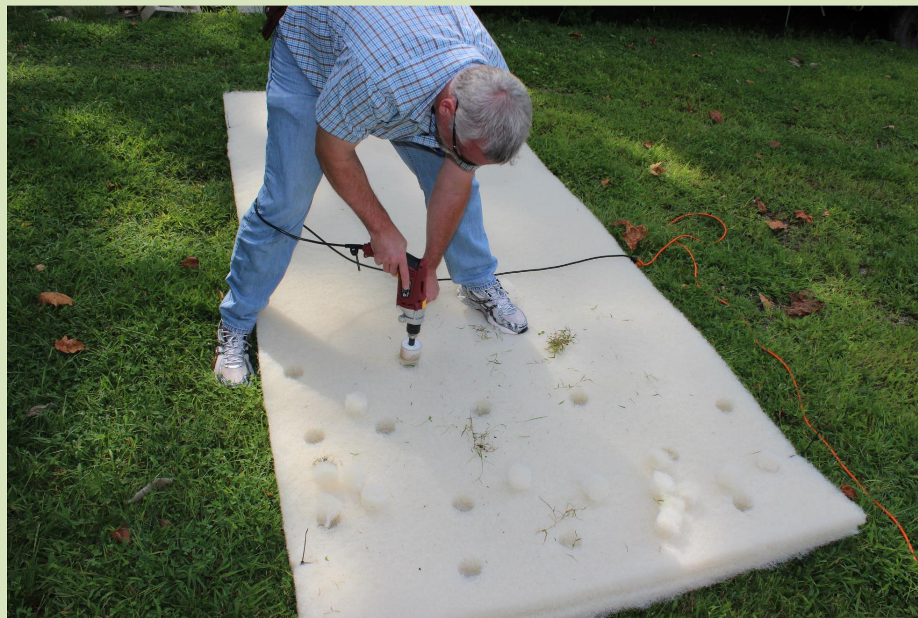
On site, drilling 2in holes for plant material.
