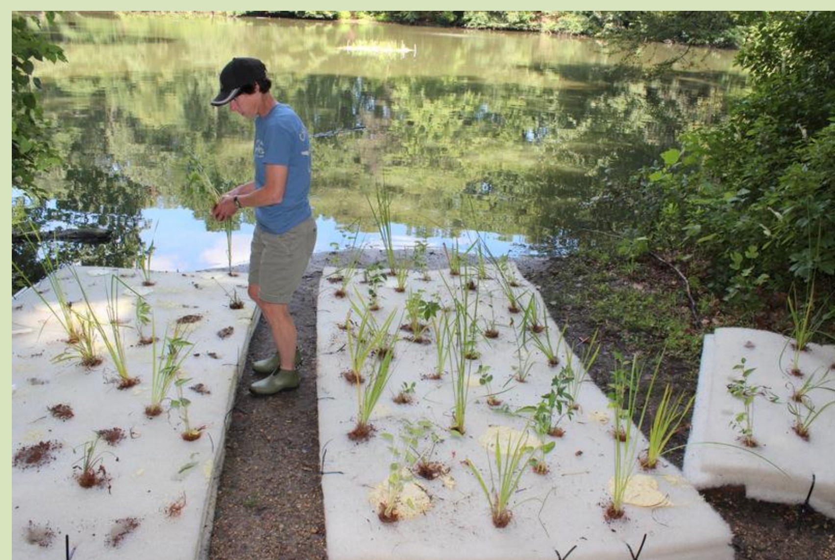
Assembling artificial floating wetlands on location.
