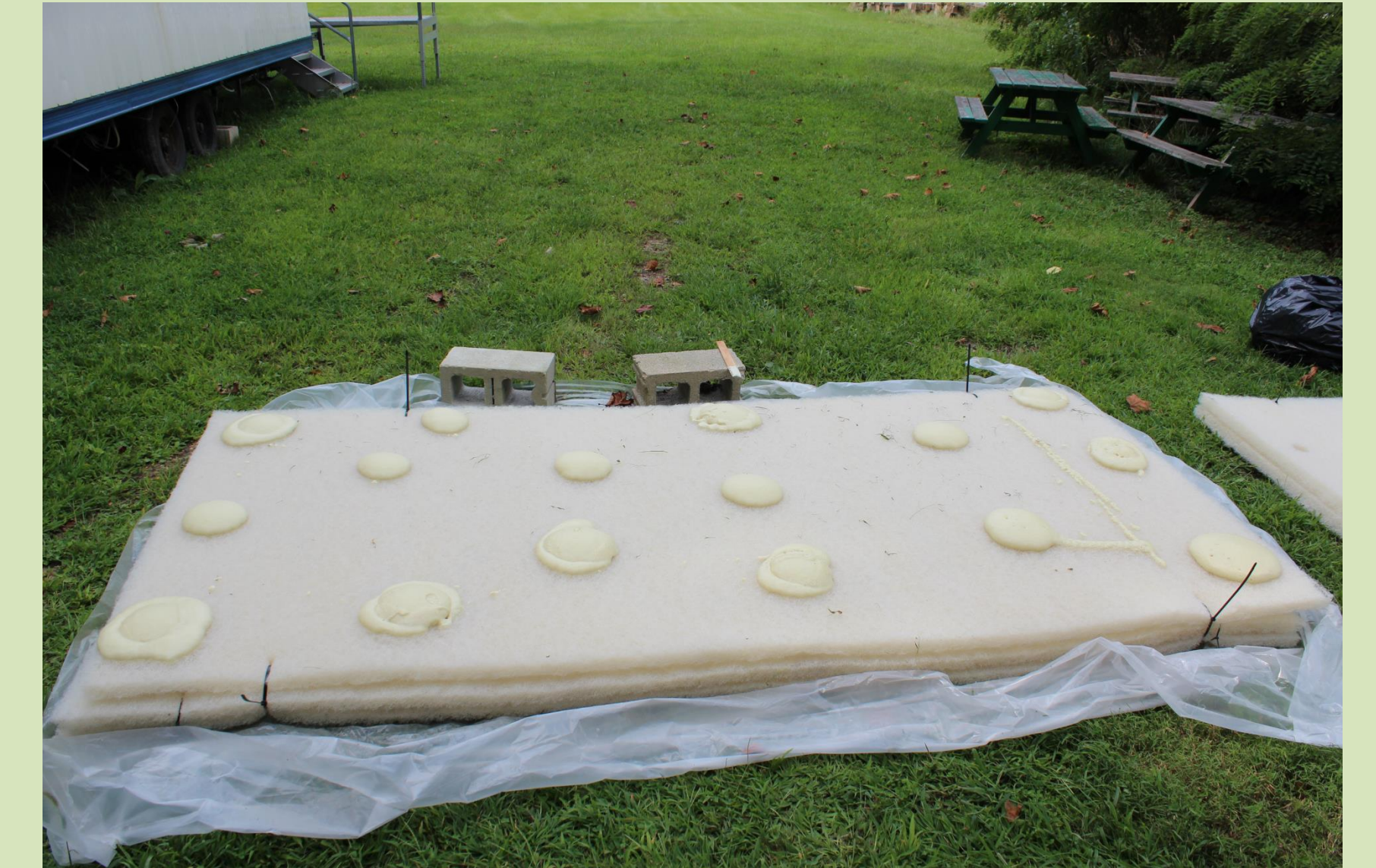
Bottom of wetland with extra foam.
